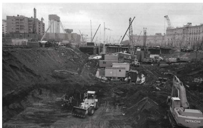
Figure 1. Construction of the tunnel with cut-and-cover method.
